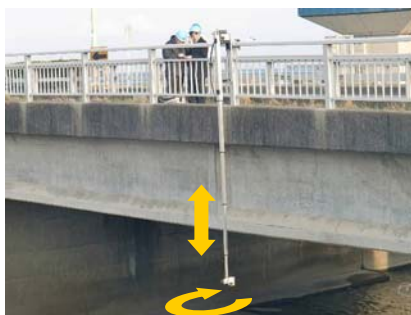
PC桁の点検
